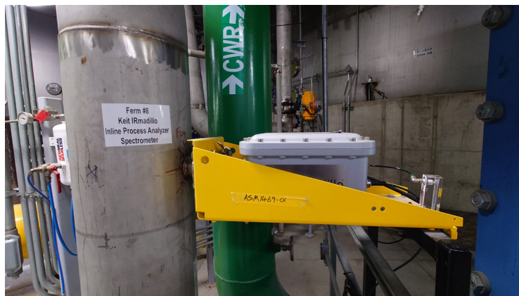
Photo: IRmadillo instrument installed in a recirculation line
