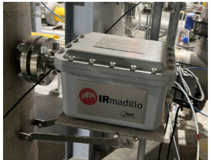
Image: IRmadillo spectrometer mounted in the recirculation loop of an ethanol fermenter
