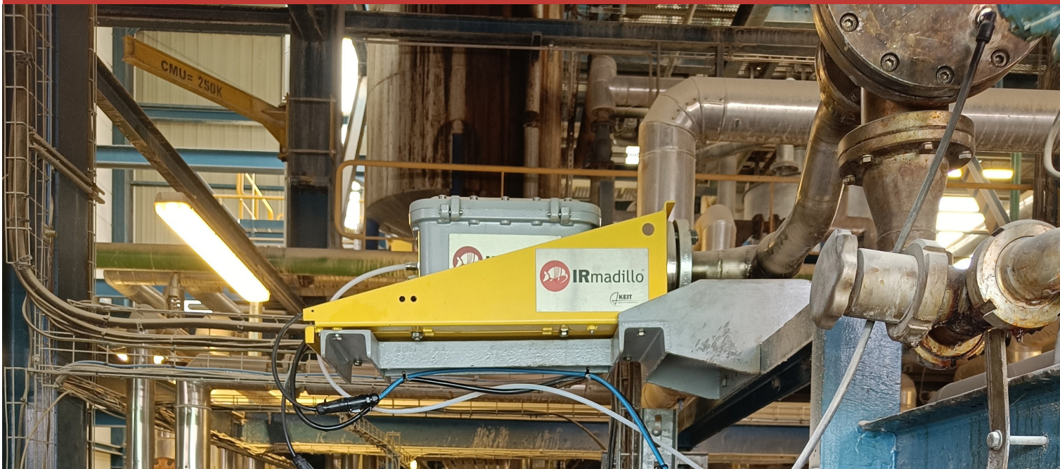
Image: Example of an inline installation of the IRmadillo in a green diesel plant
