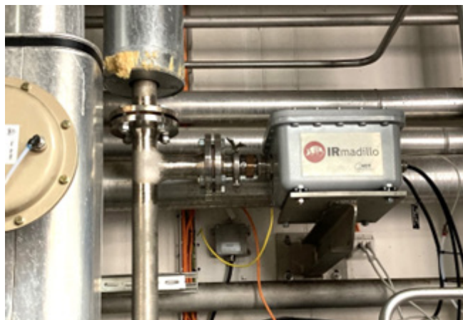
Figure 1: IRmadillo installed on the crude oil inlet
